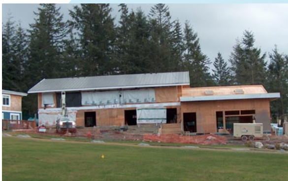
Exterior view of new wing and pool area.
